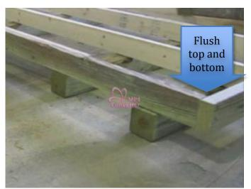
Pay special attention that the end joist is flush at the top and at the end of the frame.
