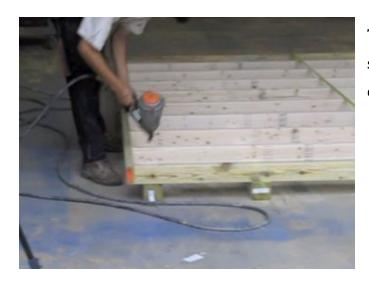
Then begin fastening to the 4x4's on the outside skids. Toenail one or two 3" nails or screws at every place where a joist meets a 4x4 skid.
