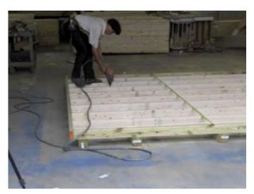
Next, place a tape measure on top of the floor joist along the middle 4x4. Be sure each floor joist is centered at the 16" mark as it is nailed to the 4x4. After the middle section is completed, finish nailing the remainder of the floor joist to the skids.
