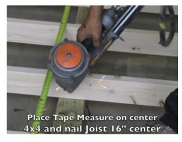
Now we are ready to nail the floor joists into the pressure treated 4x4 skids. Mark along the end where each skid should be placed
